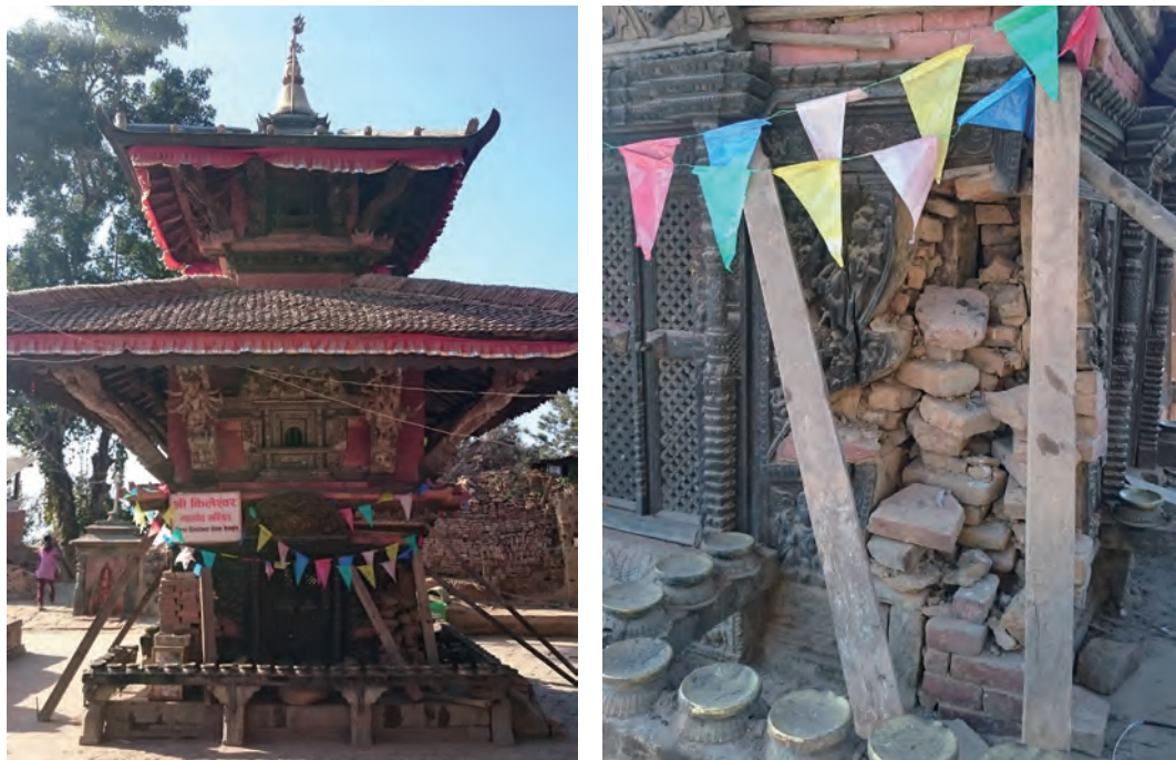
Fig.4-4 Changu Narayan Temple structure saved from collapse by the timber column
