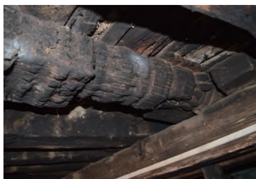
Fig.6-17 Carved pillar that was reused as a beam
