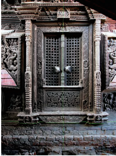
Fig.3-24 Aganchen Temple, first storey, east side (the green laser beams show the horizontal and vertical directions)
