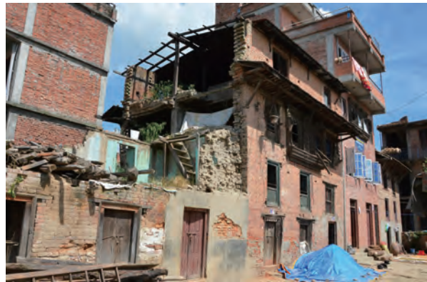
Fig.2-20 Damage situation of Khokana
