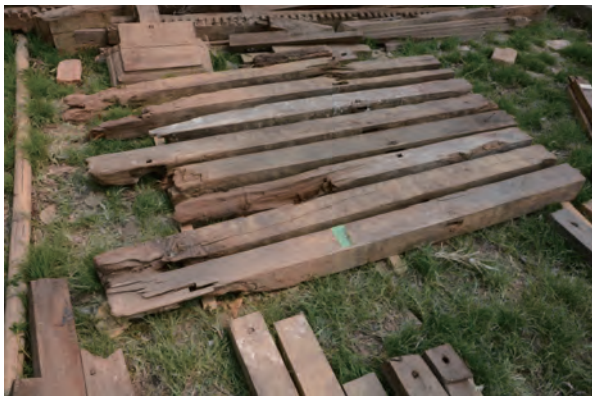
Fig.5-14 Wooden pillars around the inner brick wall of the first-story
