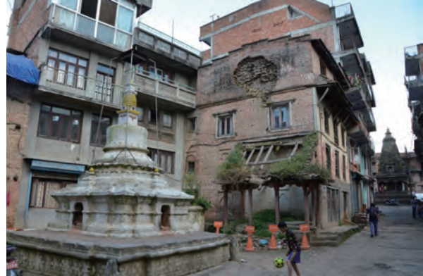
Fig.2-16 Damage situation in Kirtipur
