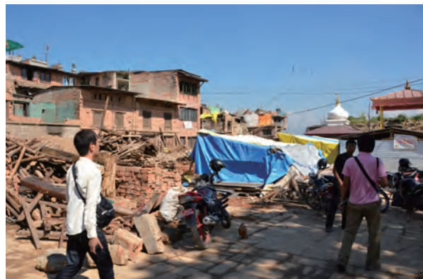
Fig.2-22 Damage situation of Bungamati
