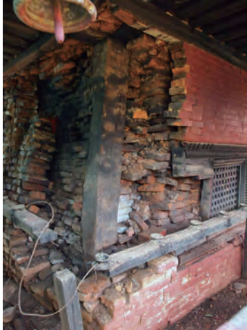
Fig.3-15 Pillar embedded into the wall at the southwest corner
