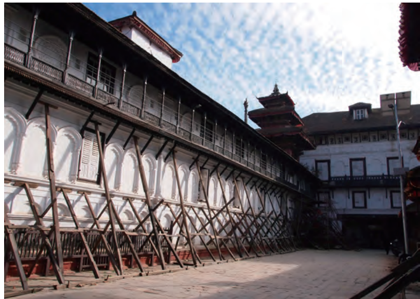
Fig.3-19 Hanumandhoka west wing façade, including the main gate
