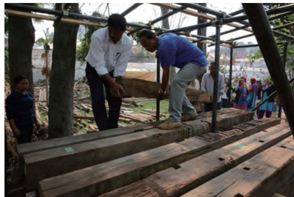
Fig.5-9 Storage of the structural members
