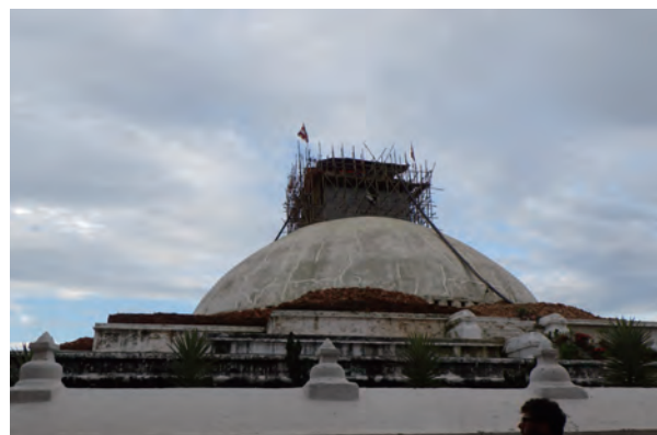
Fig.2-12 The flat top that the parasol-shaped roof was removed
