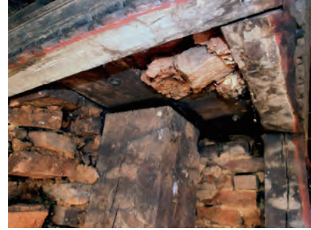
Fig.3-17 Pillar embedded into the wall, Bhairab Temple
