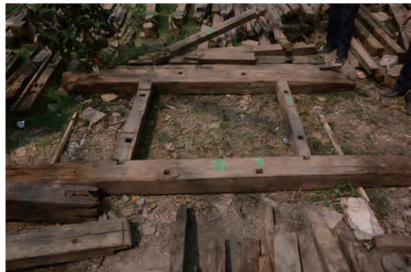
Fig.5-15 Wooden frame assumed to be a roof truss
