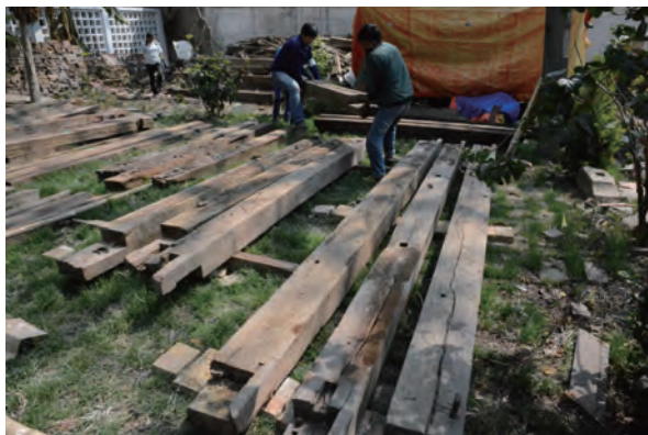
Fig.5-8 Sorting of the structural members
