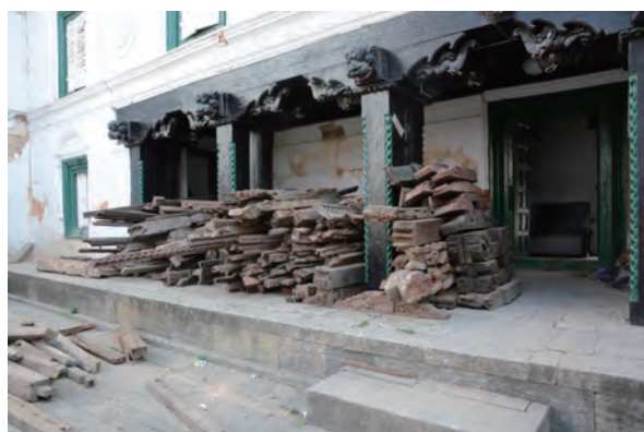
Fig.2-29 Salvaged members compiled under the porch of Dakh Chok
