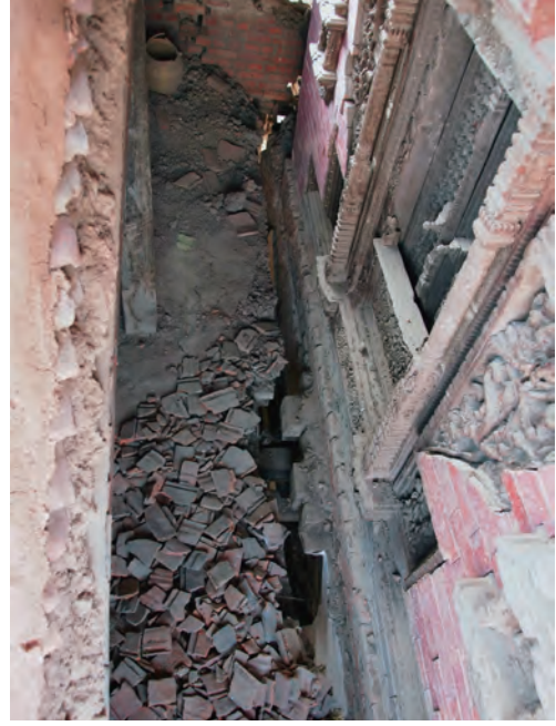
Fig.3-25 Gap between Aganchen Temple and the south wing of Mohan Chok (roof structure to the left, Aganchen Temple to the right)
