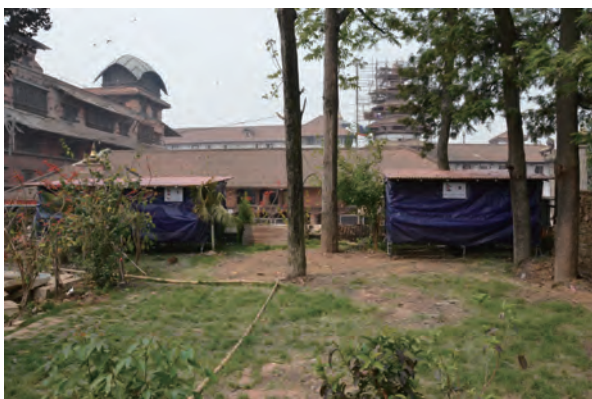
Fig.5-12 Constructed Storage facilities
