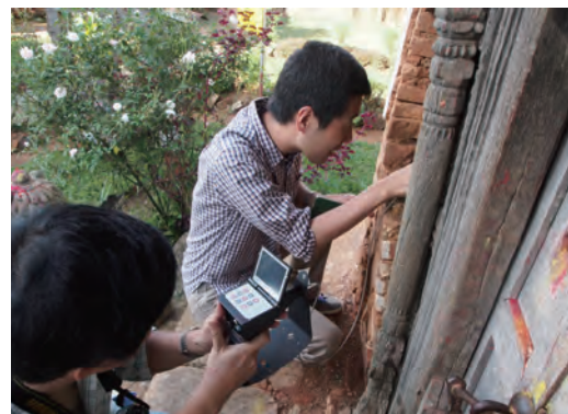
Fig.1-8 Structural survey of damaged buildings
