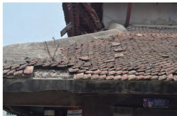
Fig.3-12 Roof tiles (Durbar Square)
