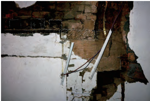
Fig.3-26 Traces on the purlins of Mohan Chok (3rd storey staircase, the white chalk marks show the section of the purlin that was cut off)
