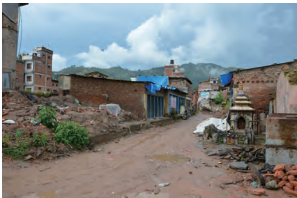
Fig.2-17 Damage situation in Sankhu
