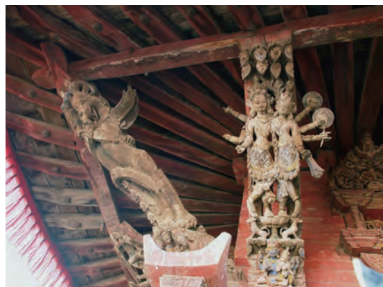
Fig.3-21 Aganchen Temple, first storey, east side (the strut to the left is kunsar)
