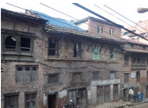
Fig.6-16 Traditional house constructed before earthquake in 1934 still remain, although the additions have been made
