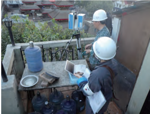
Fig.1-9 Structural survey of damaged buildings-2 (3D measurement of Hanumandhoka)
