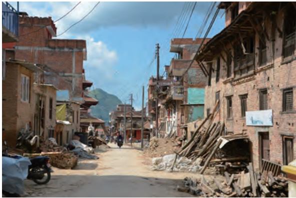
Fig.2-19 Main street in Khokana after Gorkha earthquake
