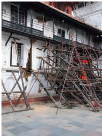
Fig.3-22 Outer west wall below Aganchen Temple
