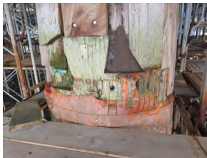
東文研で検討した材料を用いた修理(厳島神社大鳥居) Restoration work using materials evaluated by TOBUNKEN (The Torii gate of Itsukushima Shrine)
