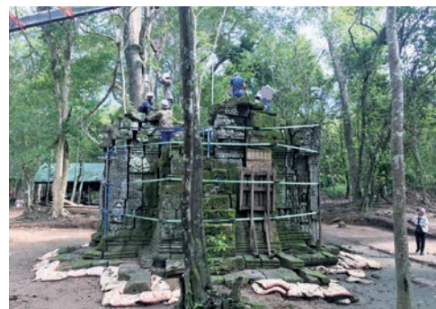
屋根の解体作業 Dismantlement work of the roof structure
