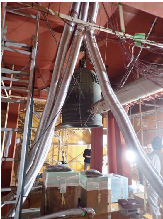
湿度制御温風殺虫処理の様子(処理空間内部) Humidity-controlled Warm-air Insecticidal Treatment
