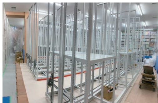
電動書架の設置 Installation of electric movable shelves
