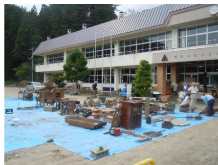
Figure 7. Emergency handling work at an abandoned elementary school, Rikuzentakata City, Iwate prefecture.
