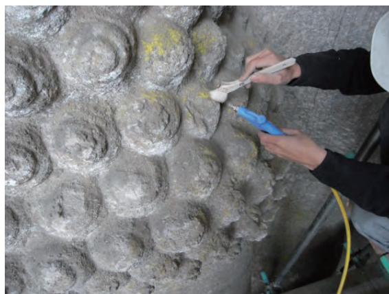
Fig.21 Cleaning epiphytes
