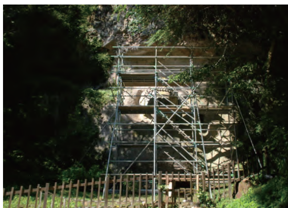
Fig.8 Scaffold at Kumano Stone Buddha
