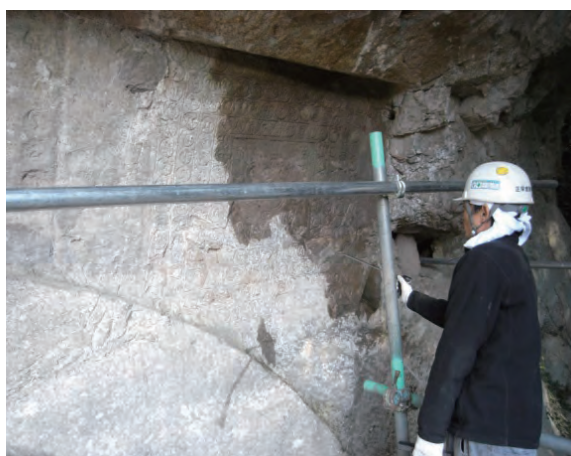
Fig.20 Applying water repellent
