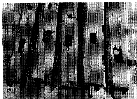
図. 29 修理柱処置後上部 Fig. 29 The upper parts of the columns after repair
