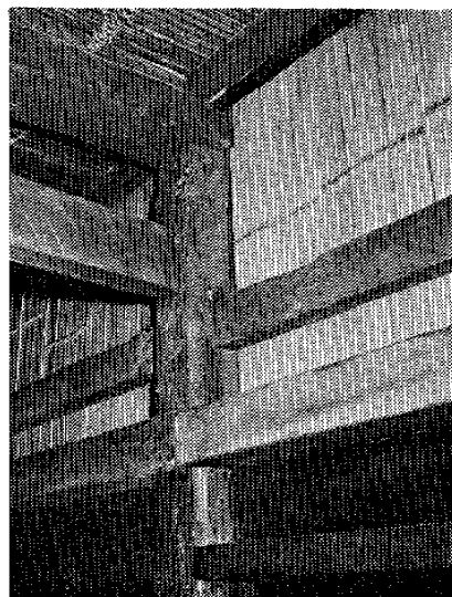
図. 31 箱木家完成後「にの十」 Fig. 31 The repaired column after reconstruction
