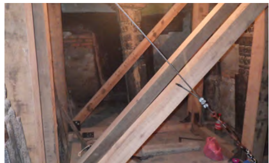
Fig.2-2-10 The stabilisation work of the inner space, below Aganchen Temple: Bracing with a wire and turnbuckles (September 2016)
