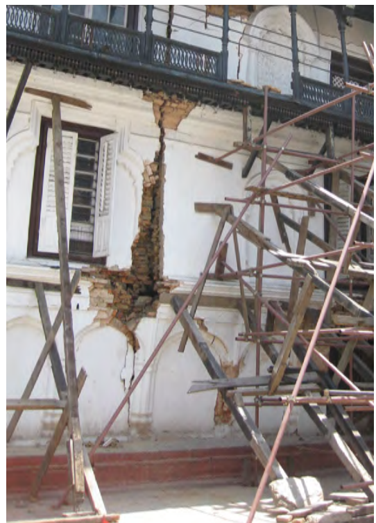
Fig.3-1-13 Gap on the outer western wall of the building below Aganchen Temple
