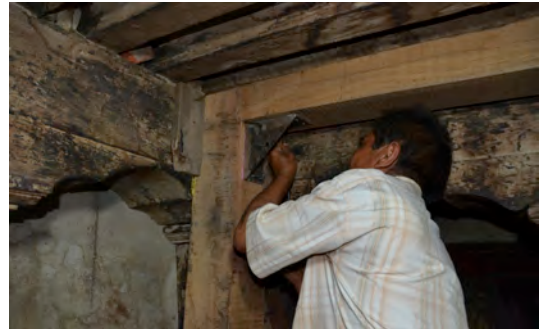
Fig.2-2-6 The stabilisation work of inner space the first storey below Aganchen Temple: Metal fitting installation (June 2016)
