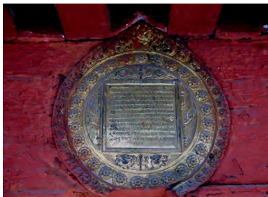
Fig.3-1-7 Inscription board indicating the data of erection of the Temple
