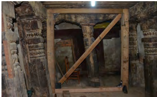
Fig.2-2-7 The stabilisation work of inner space on the first storey below Aganchen Temple: Installation of wooden frame (June 2016)
