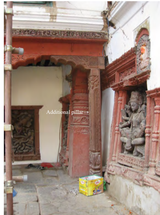
Fig.3-1-17 The column added at the western end of the north side of the south wing of Mohan Chok
