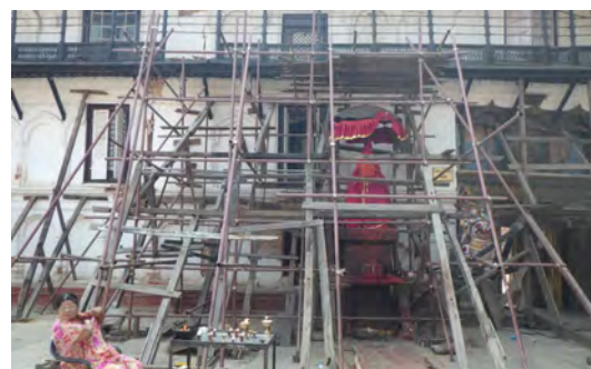
Fig.2-2-4 Before the stabilisation work (May 2016)
