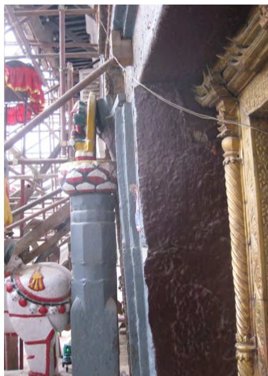
Fig.3-1-21 Inclined north gatepost of Hanuman gate
