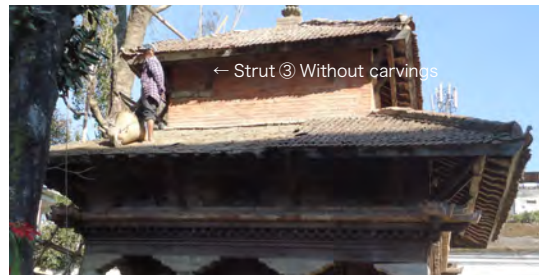
Fig.2-2-20 Photograph of the Shiva Temple during dismantling of the roof (Taken on 12 Feb. 2014, provided by ERCO)
