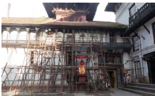
Fig.2-2-11 Completion of the stabilisation work: General view (September 2016)
