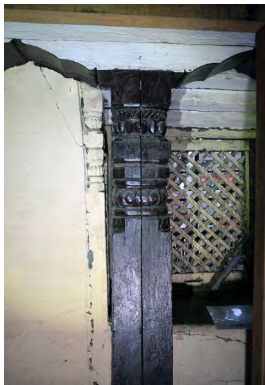
Fig.3-1-6 Western pillar and a remaining pilaster on the third storey below Aganchen Temple
