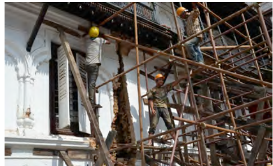
Fig.2-2-8 The stabilisation work of the exterior below Aganchen Temple: Addition and replacement of steel pipes (June 2016)
