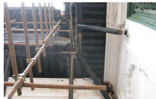
Fig.3-1-19 Balcony of the north side of south wing of Mohan Chok, view from below
