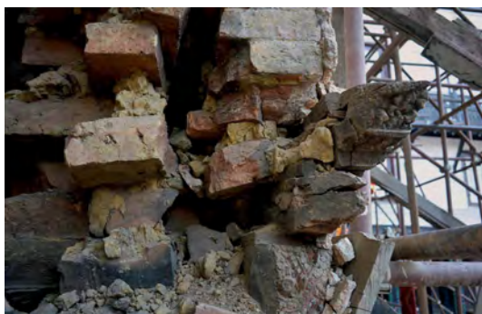
Fig.3-1-4 Cornice at the northern external corner of outer western wall on the second storey below Aganchen Temple
