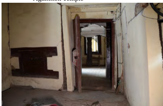
Fig.3-1-5 External south wall on the third storey below Aganchen Temple (seen from the room above Hanuman gate)
