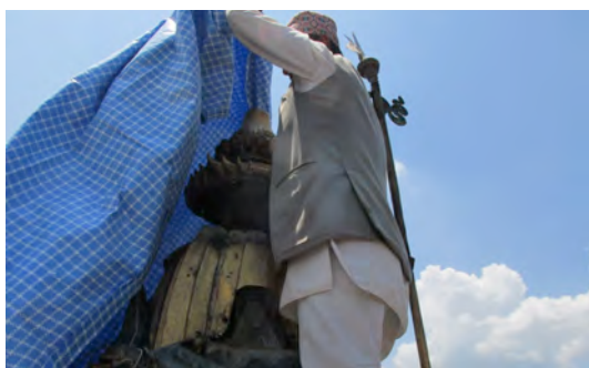
Fig.2-2-3 Waterproofing work of the pinnacle of the Aganchen Temple
