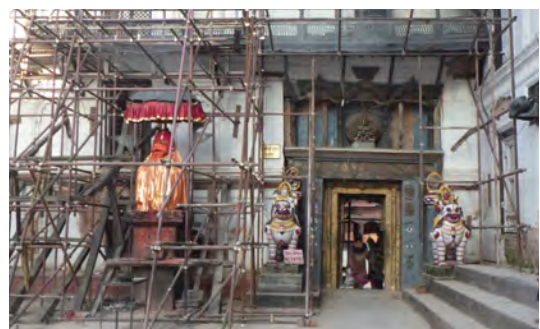
Fig.2-2-12 Completion of work: Gate front was organised (September 2016 )
