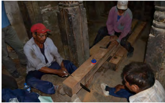
Fig.2-2-5 The stabilisation work of inner space on the first storey (the ground floor) below Aganchen Temple: Wood-processing work (June 2016)
