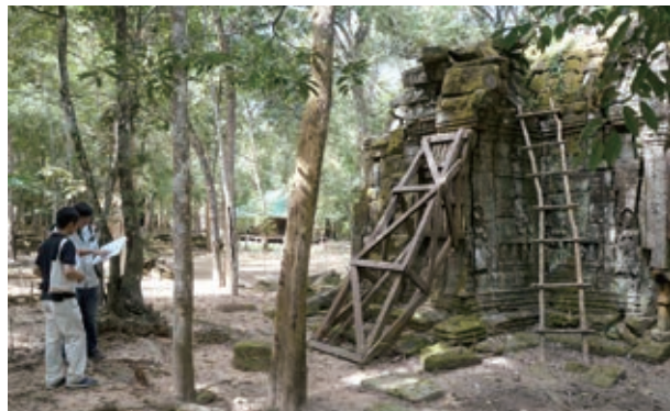
支保工の現状調査 Survey of the current condition of the temporary supports
