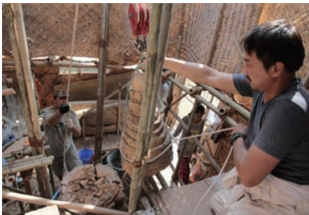
被災した尖塔部分の解体修復 Dismantling and restoring of a damaged spire
