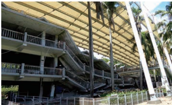
921 地震教育園區内の被災した光復國民中學の展示 Damaged Guangfu Junior High School exhibited in the 921 Earthquake Museum of Taiwan
