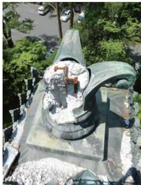
*Left: Survey with the cherry picker. The bronzed black kite that had fallen from the pedestal is evident at the bottom right. Right: The damaged bronze adornment and top of the pedestal. The stone leaves blossoming from the pedestal's center are barely restrained by a loosened bolt.*
