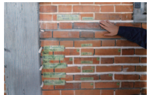
国宝・旧富岡製糸場 目地試験施工の状況 Experimenting joint materials at Tomioka Silk Mill, a national treasure
